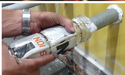
Gluing TBA Firefly Penowrap to substrate
