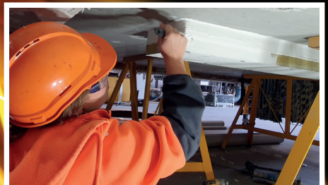
Buttering Up The Edges Of The TBA Firefly Intubatt
